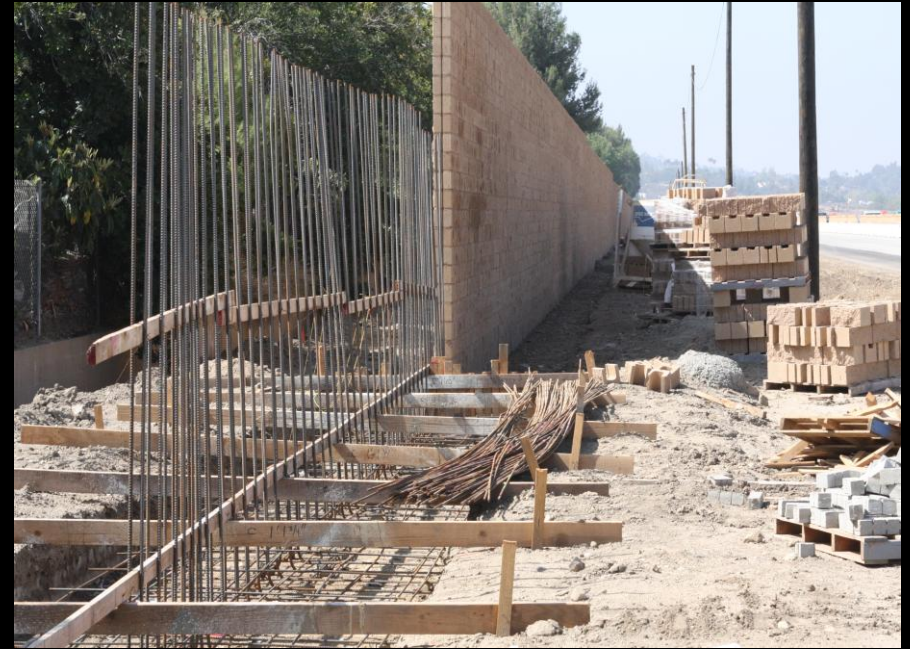
Rebar, foundation, and block work
